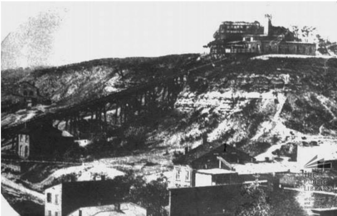
Looking north from Pendleton/Over-the-Rhine at the Mt. Auburn Incline with Christ Hospital shown at the top of the hill. The incline was built in 1872 and its right of way remains as a public stairway.
